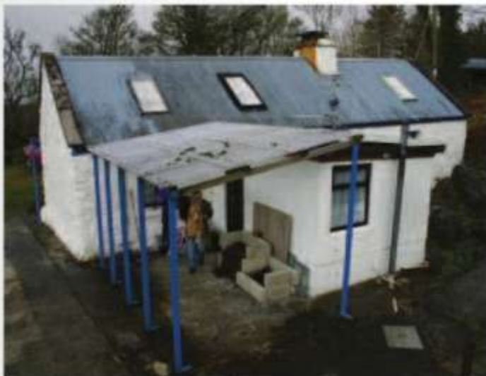
The existing cottage originally had a glazed covered area to the south which the clients enjoyed sitting under on the occasional dry Mayo day!
